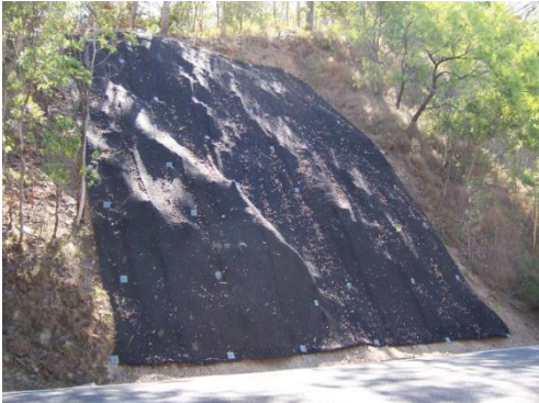
Soil Nailing & Mesh Slope Stabilisation – Cairns
