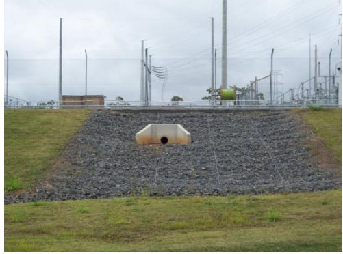
Rock Mattress Outfall Protection – El Arish
