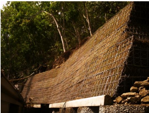
Mechanically Stabilised Earth Wall – Whitsundays
