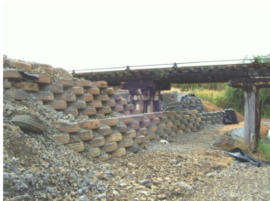
Ecoflex Retaining Wall for Hardstand – Daru Ck
