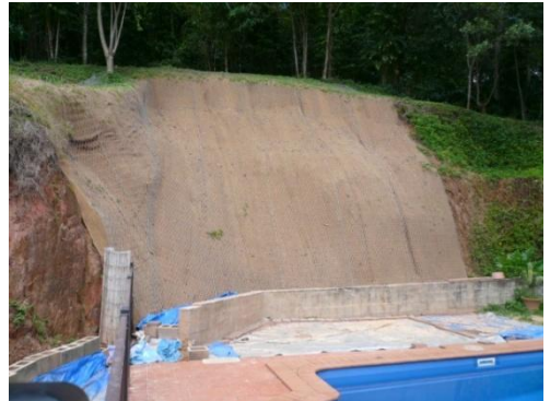
Soil Anchors & Mesh Slope Stabilisation – Cairns
