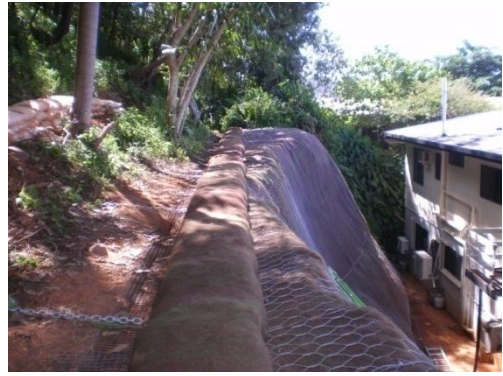
Slope Stabilisation Anchors & Mesh – Cairns
