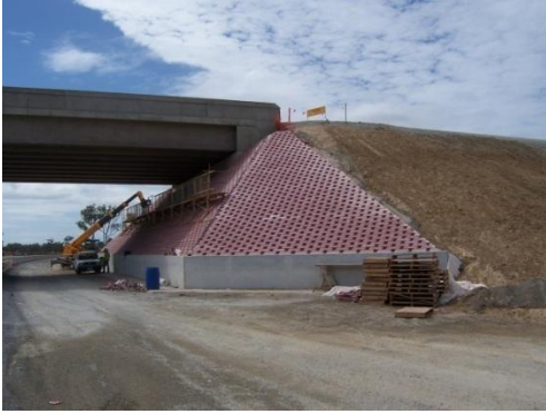
Abutment Protection -Townsville Ring Road
