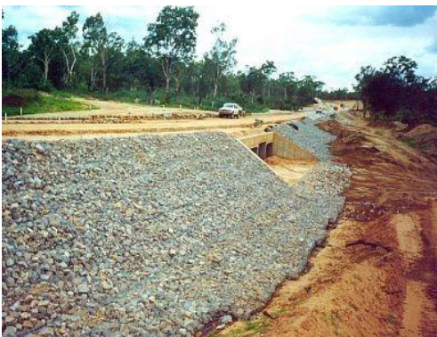
Rock Mattress Scour Protection – Townsville
