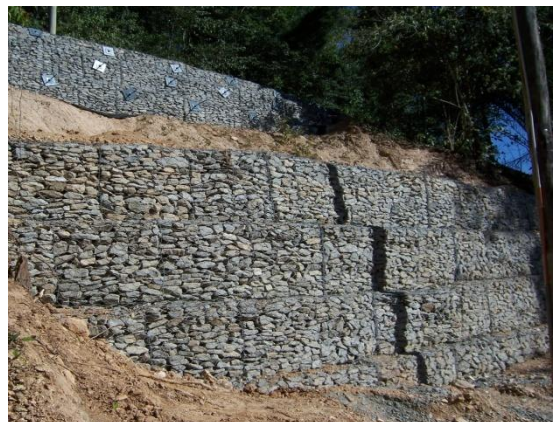
Soil Nails and Gabion Wall - Mossman
