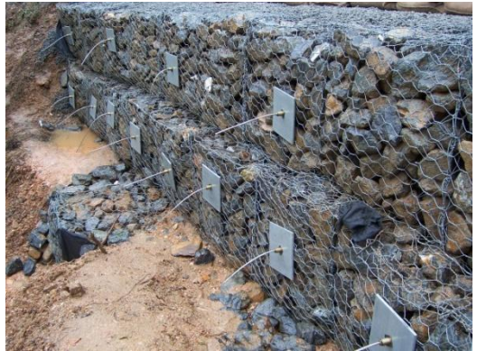
Soil Anchors & Gabions – Gillies Highway
