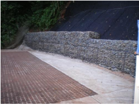
Gabion & Mesh Slope Stabilisation – Cairns
